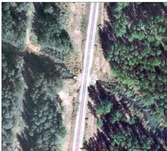
Figure 6. Incision through a road prism. The optical imagery at the left shows a road prism with through-going culvert. As seen in the shaded-relief image below left, the road prism appears as a dam to flow in the channel. A short line segment is digitized between the two ends of the culvert, and the DEM is incised along this line.
